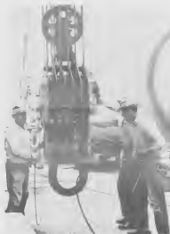
THE BLOCK, clearly showing the thirteen strands of the lead line, is ready to raise the 100-ton load.
